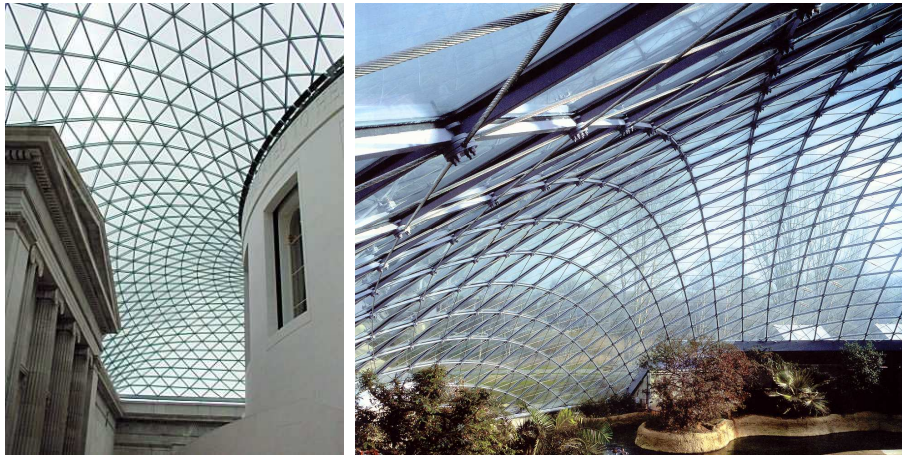
Fig. 2. Left: Triangulated truss shell structure consisting of bars and joints (Great Court, British Museum, London). Right: Hybrid type of structure consisting of a quad-rangular truss stabilized by pre-stressed diagonal cables (Hippo House, Berlin Zoo)
